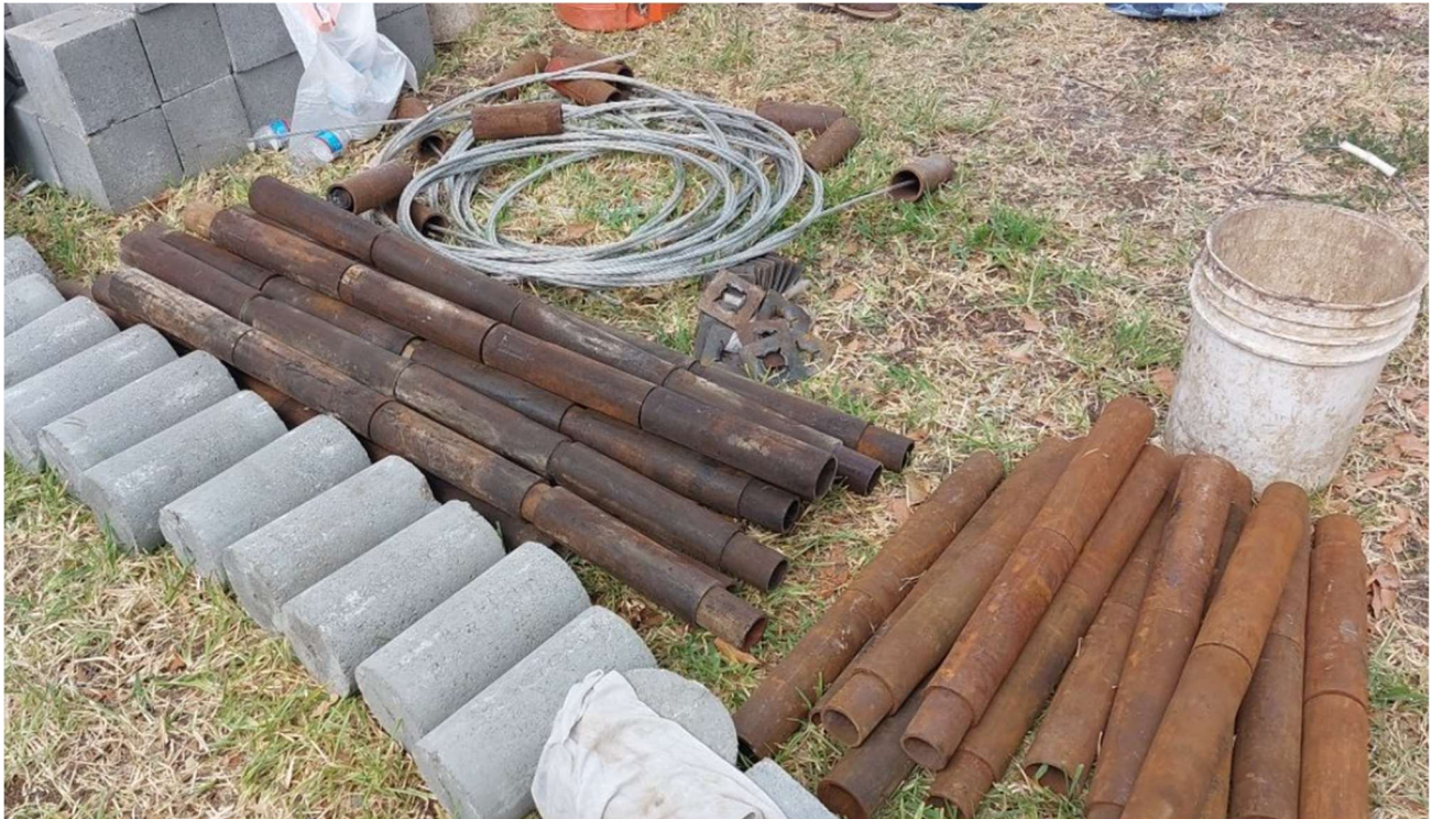
Piling Components at 16121 Wall St (Jersey Village, TX)
