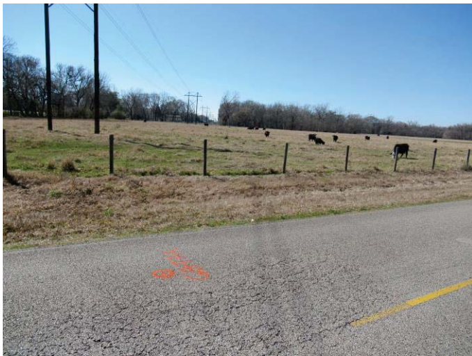
Moderate to severe alligator cracks along CR 30 near boring GB-GB-77A
