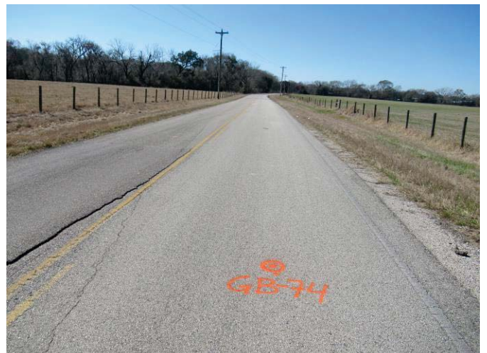
Longitudinal cracks near overlay section of pavement along CR 30 near boring GB -74
