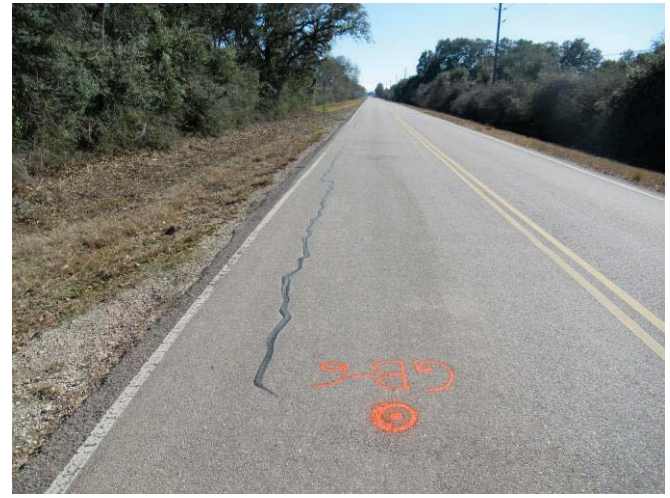
Minor Edge Cracking and patching along CR 25 near boring GB-6
