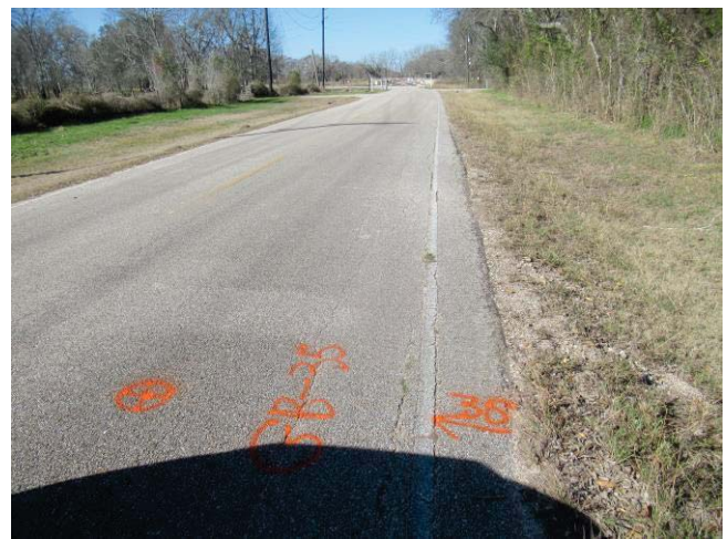
Minor longitudinal cracks and rutting along wheel path near boring GB -35 along CR-34
