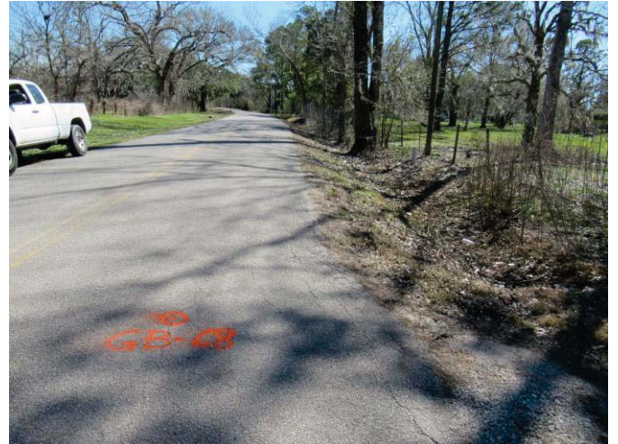
Minor joint and edge cracking near driveway intersection along CR 671 pavement near GB-68
