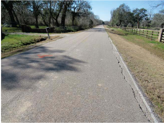
Moderate to severe edge cracking with pavement settlement near boring GB-19 along CR 36
