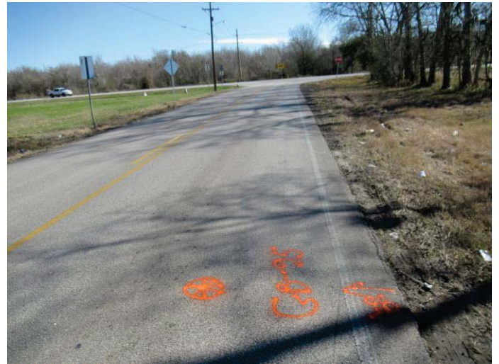
Minor fatigue cracks with edge settlement along CR 30 near boring GB-95
