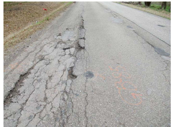
Severe fatigue and edge cracks due to lack of edge support/subgrade settlement along CR 30 near boring GB-85
