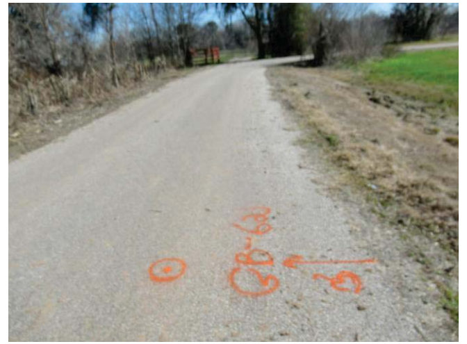
Minor distresses with loss of subgrade support along the edges of CR 612 near boring GB-62
