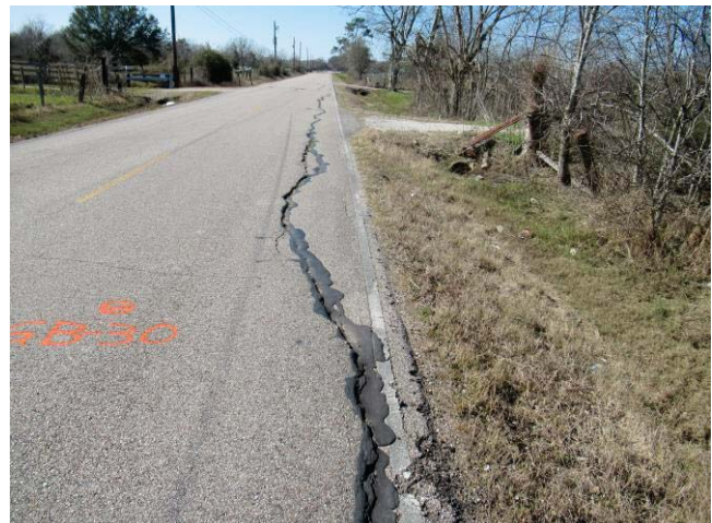
Deep longitudinal Cracks along the edges of the road with no edge support near GB-30 along CR 36
