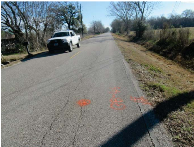
Existing roadway and ditch with longitudinal cracks along CR 34 near boring GB-46.
