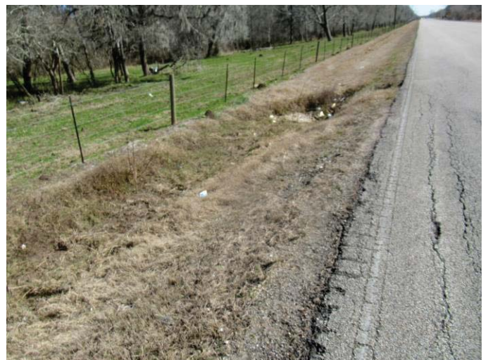
Longitudinal and edge cracking along CR 30 near GB-88 with settlement due to loss of subgrade.
