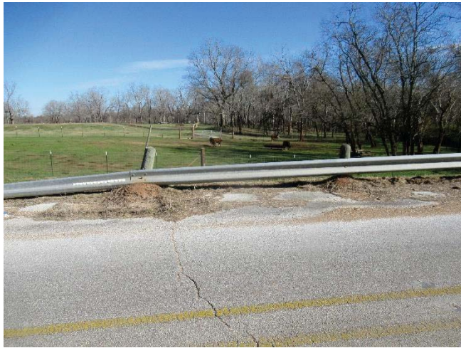
Transverse crack along CR 34 before the bridge crossing location near boring GB-40
