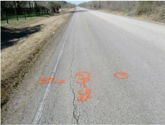
Longitudinal cracks on the onset of alligator (fatigue) cracking along CR 30 near boring GB-GB-93
