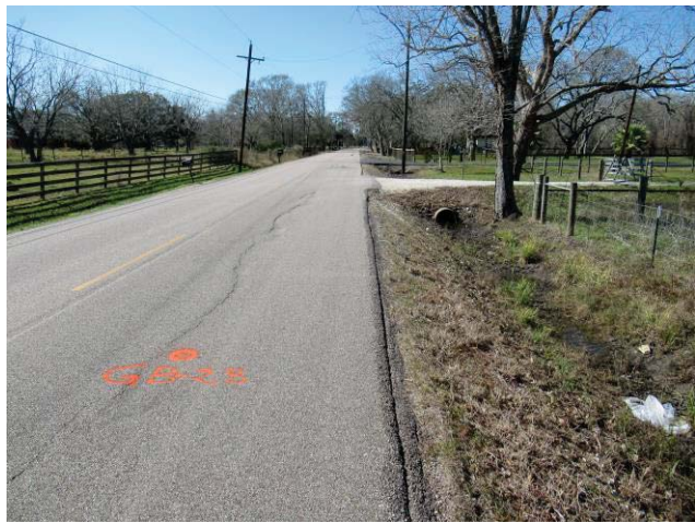
Moderate to severe longitudinal cracking with visible overlay layers near boring GB-28 along CR 36
