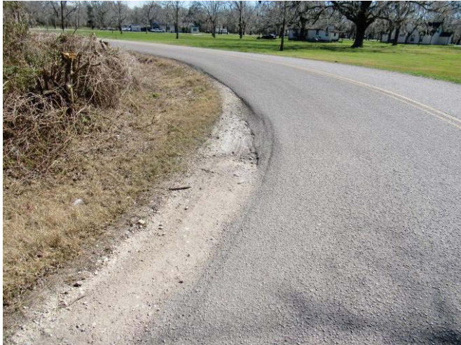
Minor distresses with pavement settlement with lack of edge support near boring GB-66 along CR 671
