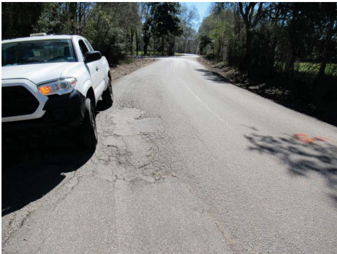
Severe alligator cracks and potholes repaired and patched near boring GB-69 along CR 671
