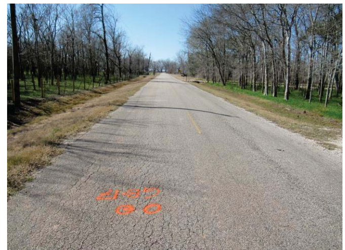
Longitudinal cracks on the onset of alligator cracking on the longitudinal joints near GB-17 along CR 36
