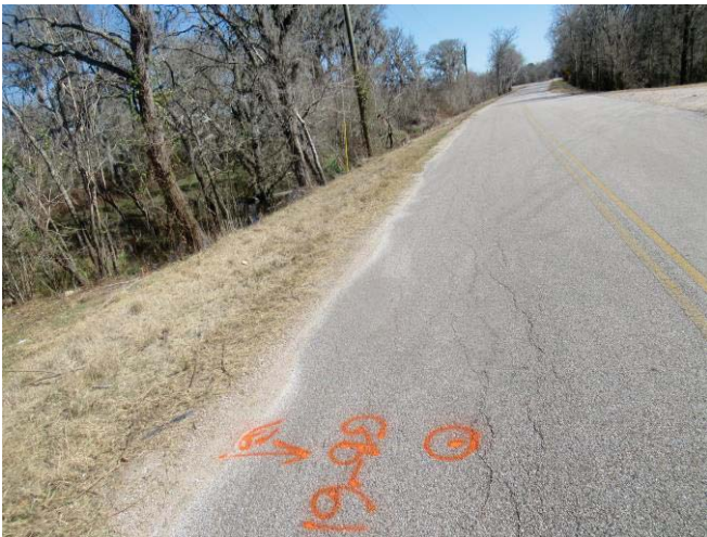
Longitudinal and fatigue cracks along CR 611 near boring GB-61 with elevated pavement shoulders
