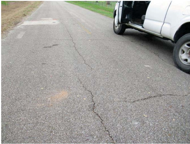
Block cracking along CR 611B near boring GB-56
