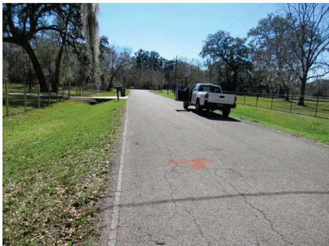
Block cracking along CR 611A near GB-54 which is a combination of longitudinal and fatigue cracks.
