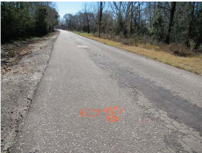
Severe alligator cracks and potholes repaired along CR 518 near boring GB-63
