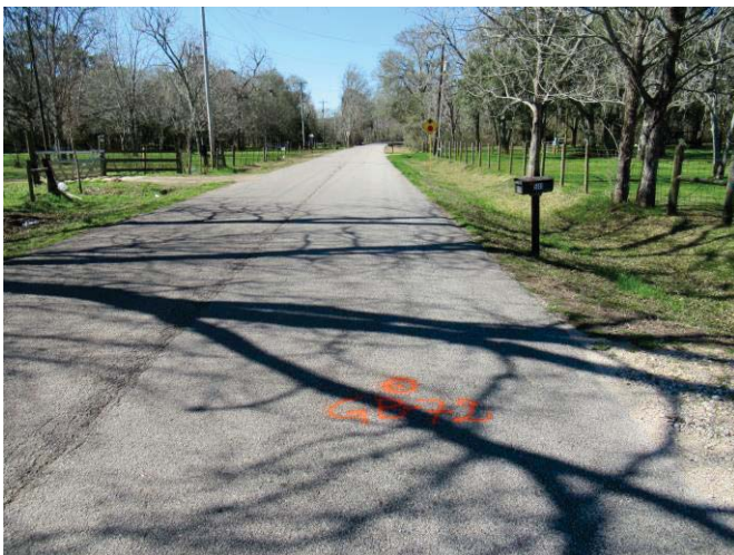
Fatigue and joint cracks at overlay sections of pavement along CR-30 near boring GB-72
