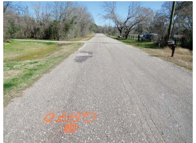
Severe fatigue & longitudinal cracks with visible potholes, repair patches near GB-70 along CR 670
