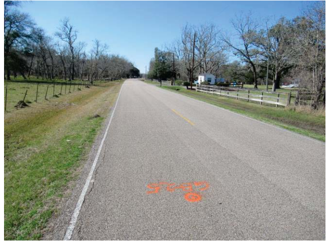
Minor longitudinal edge cracking with polished aggregate along CR 36 pavement near GB-25
