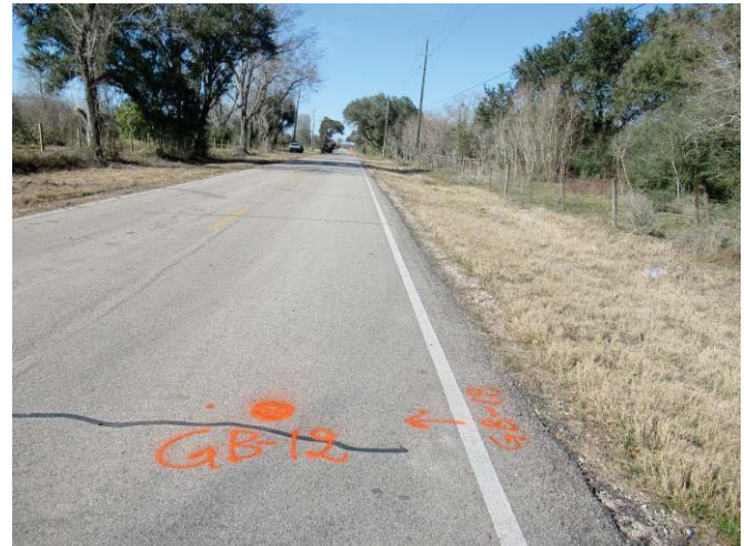
Minor transverse cracks with patching along CR 25 near boring GB-12
