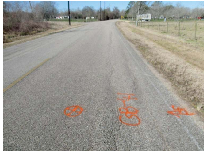
Longitudinal cracks with raveling and visible settlement of pavement along CR 34 near GB-41
