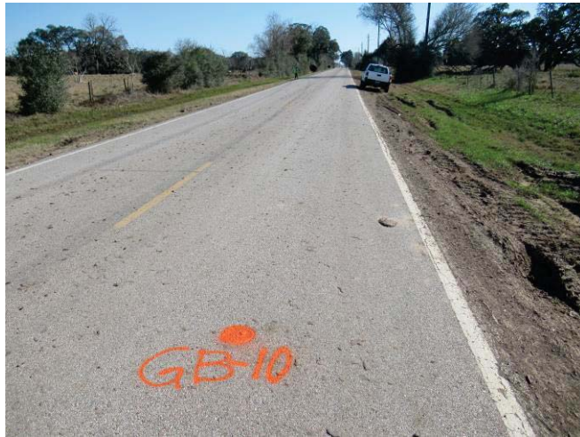
Existing roadway and ditch with minor distresses along CR 25 near boring GB-10.
