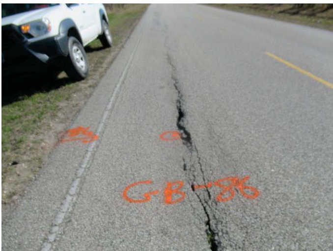
Severe longitudinal crack seen near GB-86 along CR 30 causing moisture infiltration & roughness.
