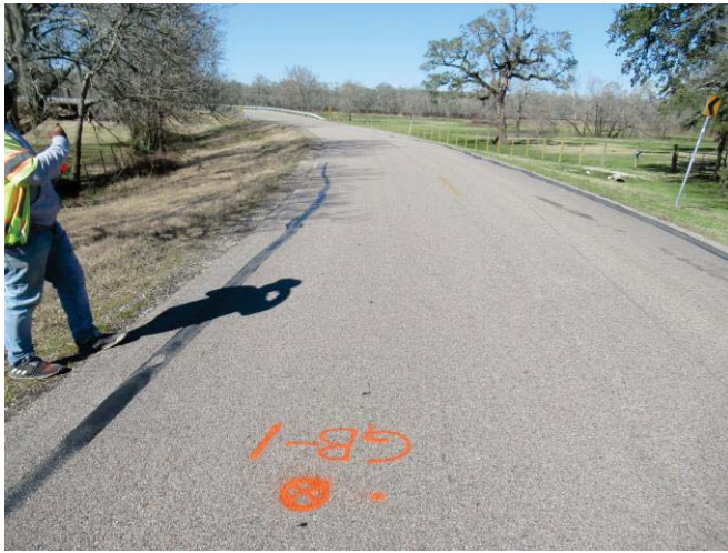
Edge Cracking with patching due to subgrade failure along CR 25 near boring GB-1
