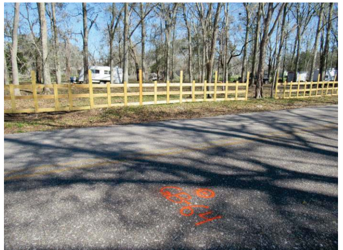
Severe polished aggregate with minor bleeding on half width of pavement near GB-64 along CR 518
