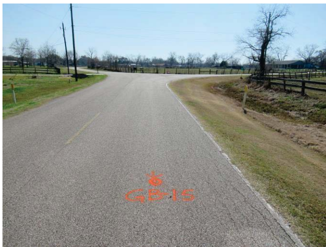
Fatigue and Edge Cracking along existing roadway along CR 36 near boring GB-15
