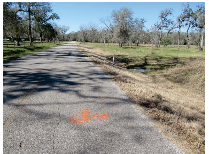
Minor longitudinal cracks along CR 611A near GB-55 with minor pavement stripping.
