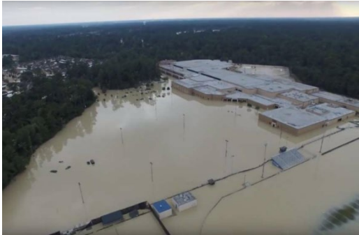
Harvey Flooding at Kingwood High School
